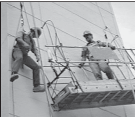
On single-point and two-point adjustable suspension scaffolds, workers must be protected with guardrails and personal fall-arrest systems.
